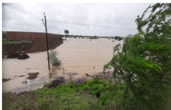
Encroachment and flooding in the Vena River
